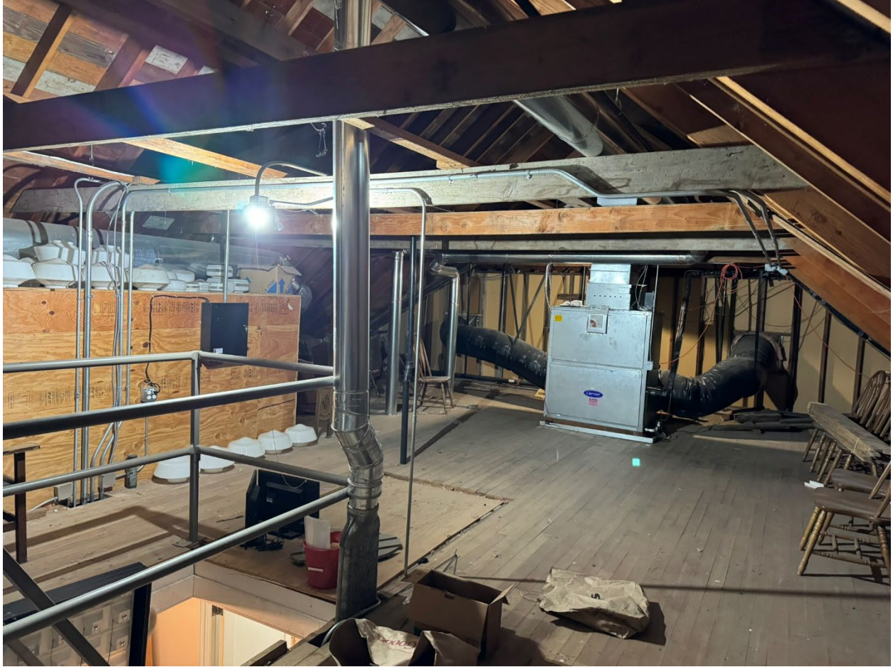
Community center - Attic
