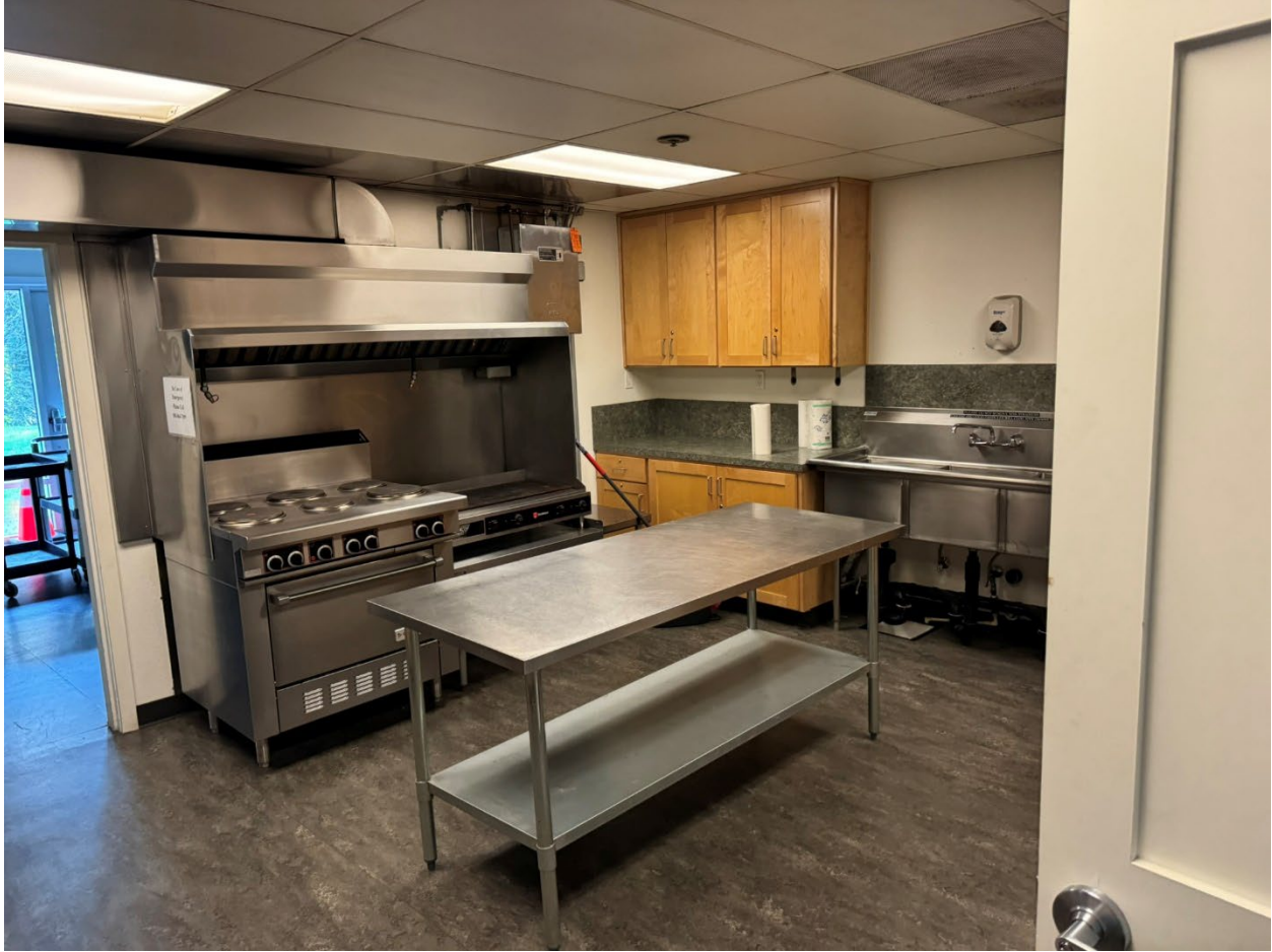
Community center - kitchen in downstairs
