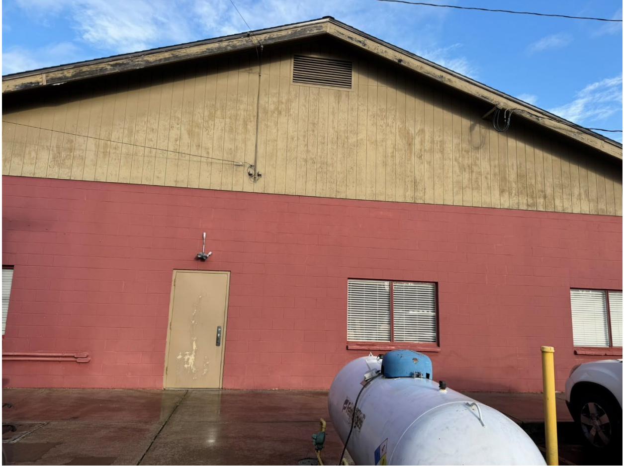
Annex – Side facing northeast
