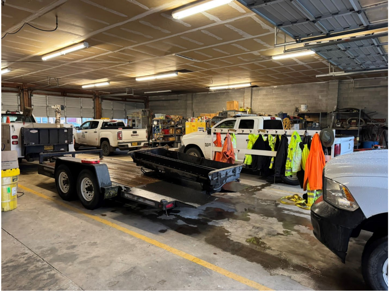
Annex - Garage bays on east side of building facing Ferry Street
