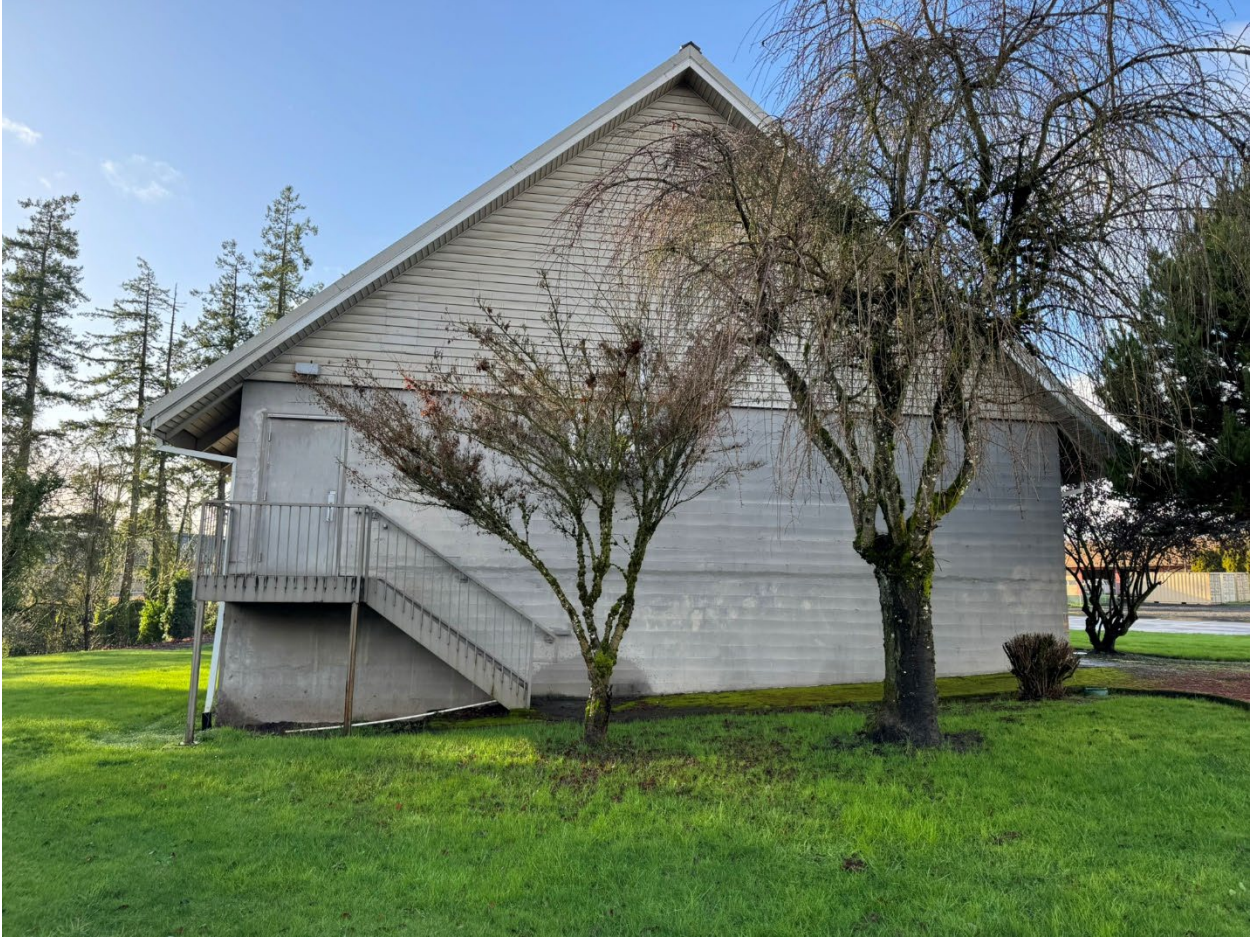
Community center – Side of building face west
