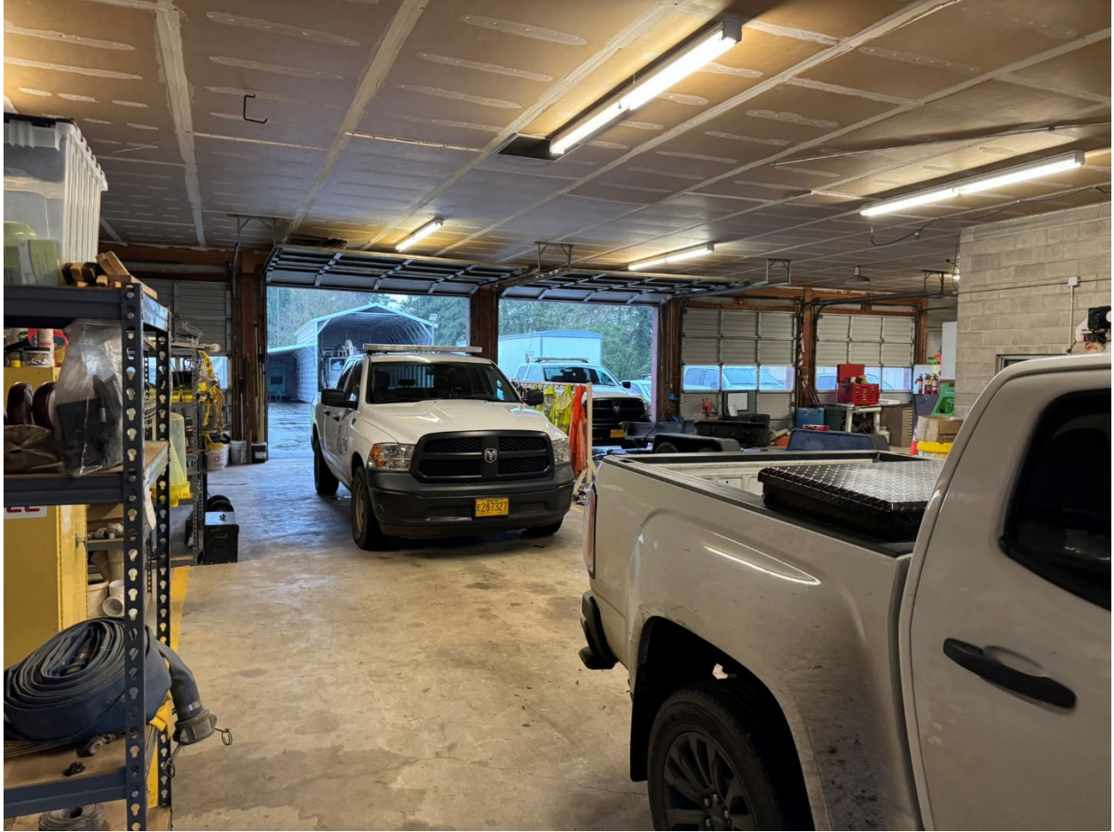
Annex - Garage bays on east side of building facing building rear
