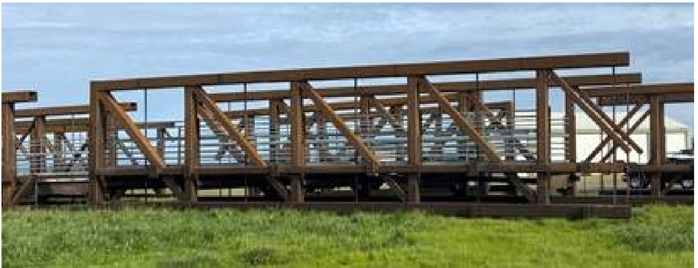
The 220-foot steel midspan replacement before it is assembled and craned over the Yamhill River and attached to the concrete abutments. It weighs approximately 225,000 lbs.
