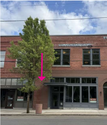
Control joint at Harris and Stuckey Buildings
