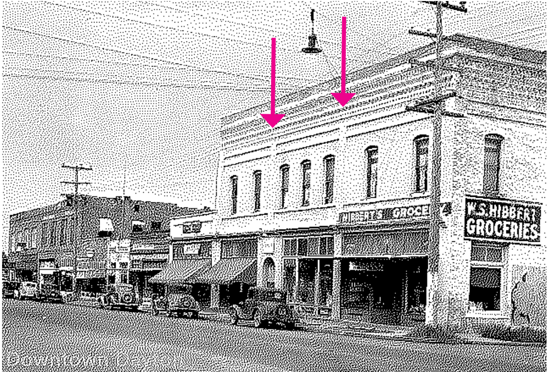
Brick detailing creating bays at the old Opera House
