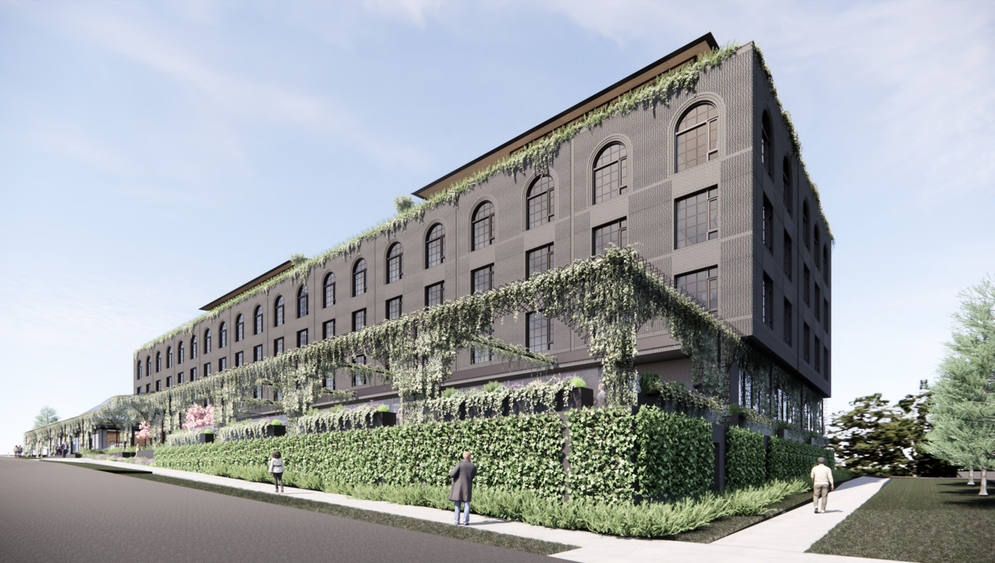
View from 2nd & Ferry Street
