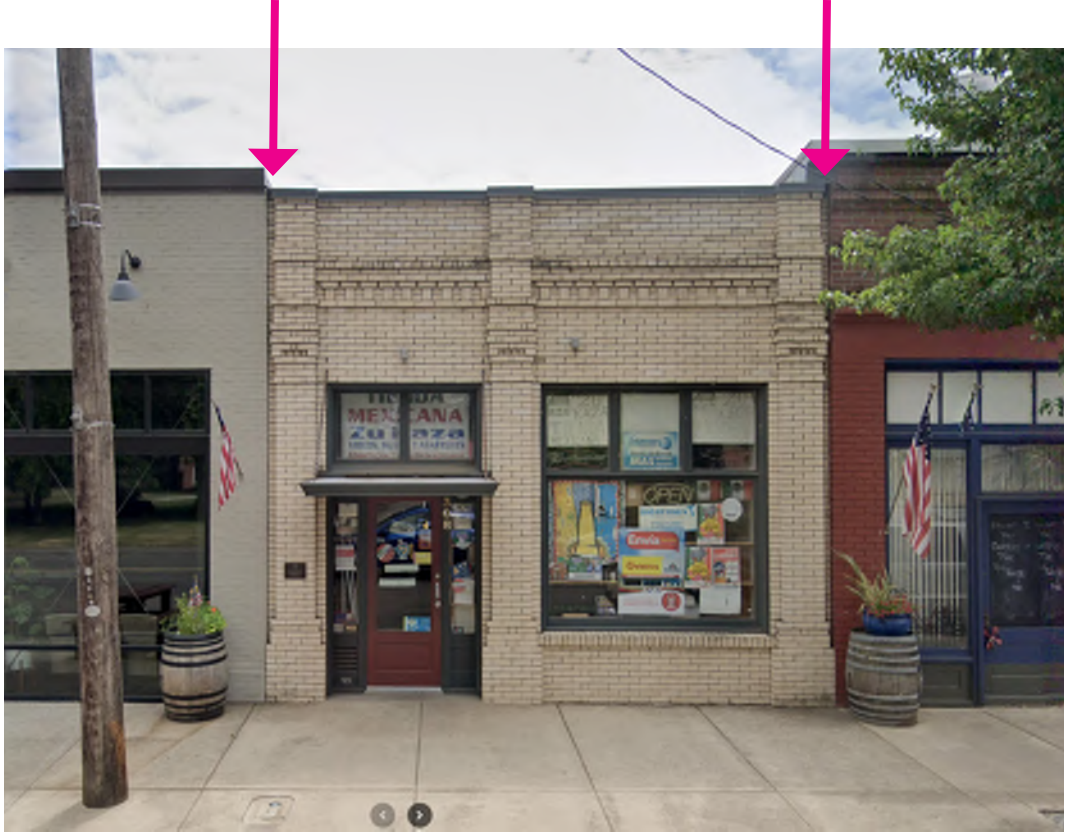
Brick detailing at Tienda Zu Kaza
