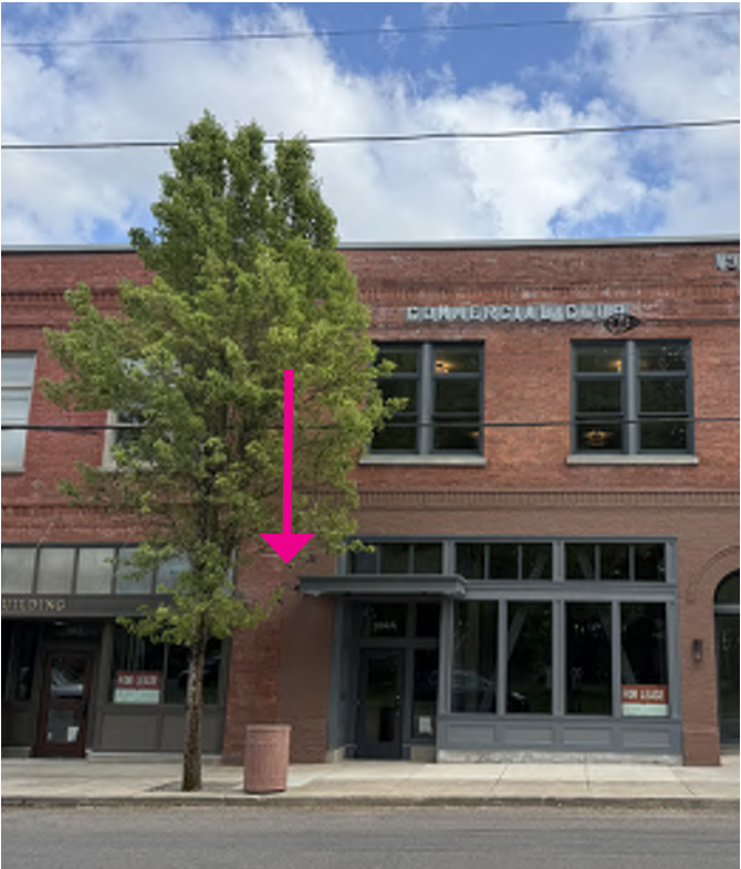
Control joint at Harris and Stuckey Buildings
