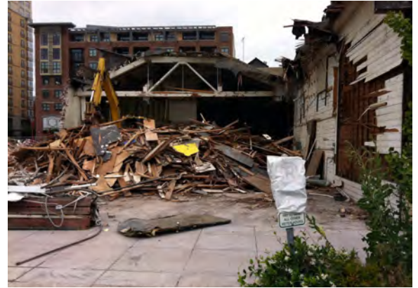
Demolition of a contributing building, 2011
