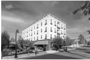
Atticus Hotel - McMinnville - 4 stories - 55 feet
