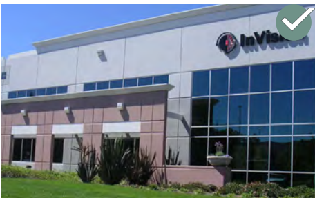
Articulating walls with architectural details, and window moldings help achieve a sense of human scale in this industrial context.
