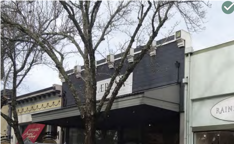
In Downtown commercial development, design a roof to be visually subordinate, and to be concealed behind parapet walls.
