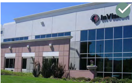
Articulating walls with architectural details, and window moldings help achieve a sense of human scale in this industrial context.
