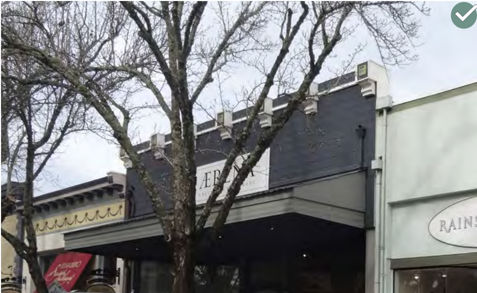
In Downtown commercial development, design a roof to be visually subordinate, and to be concealed behind parapet walls.
