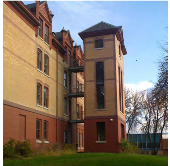
New construction on the Oregon State University campus provides additional egress to the historic building.
