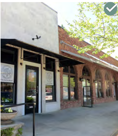
Use an accent material to highlight an important feature such as an entry or window.
