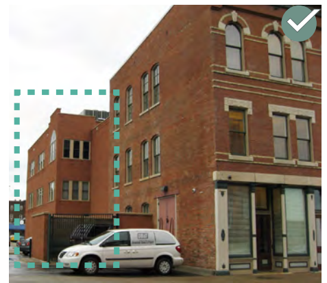
Where possible, locate a building addition to the rear of the existing structure.
