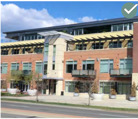
Step back a larger building mass from the street to reduce looming effects.
