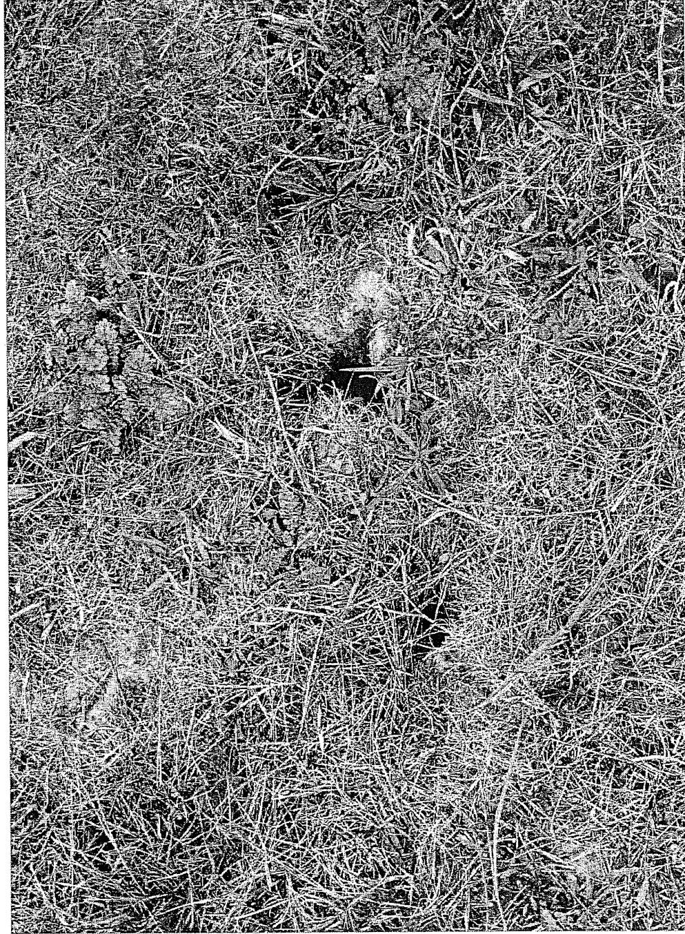
Photo 3. Typical animal burrows and desiccation cracks.
