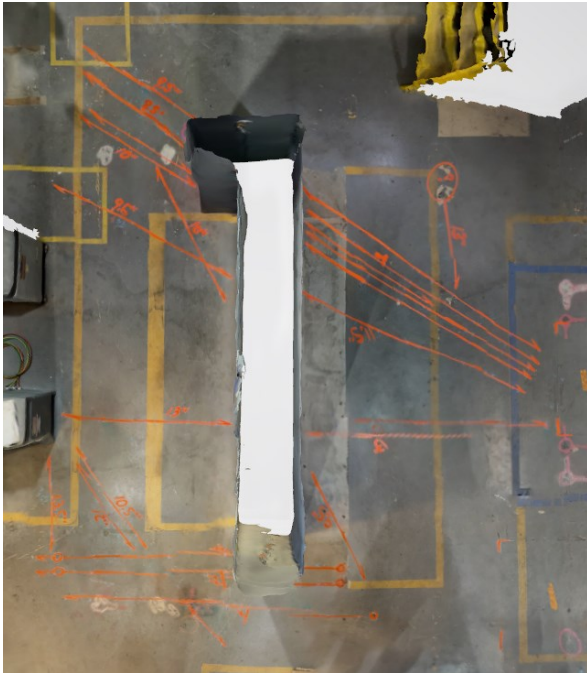
Samples of Concrete GPR work at a current airport project, as captured with 3D LIDAR at time of service.
