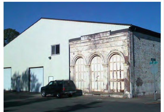
An 1860s Harrisburg building is swallowed up—literally!
