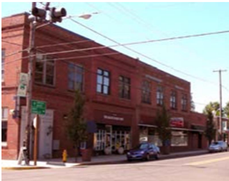
Figure 4. Ferry Street between 3 rd and 4 th
