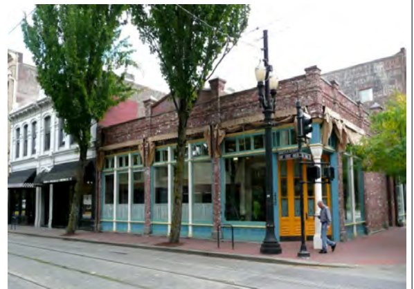
The Freimann Building in Portland is a successful reconstruction based on thorough documentation.
