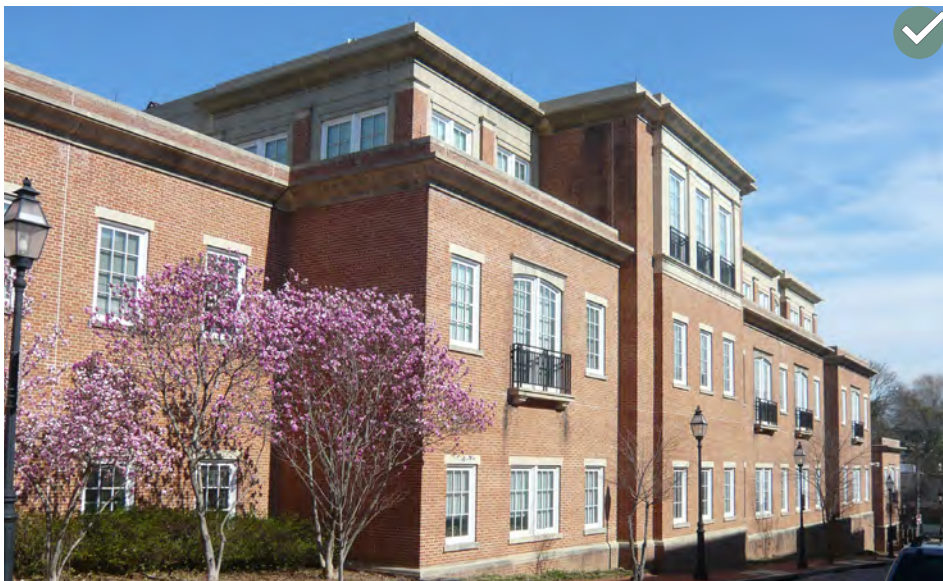
Use vertical articulation techniques to add visual interest and reduce perceived mass.
