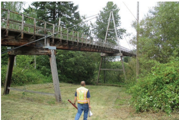
Jared inspecting the bridge in 2013.
